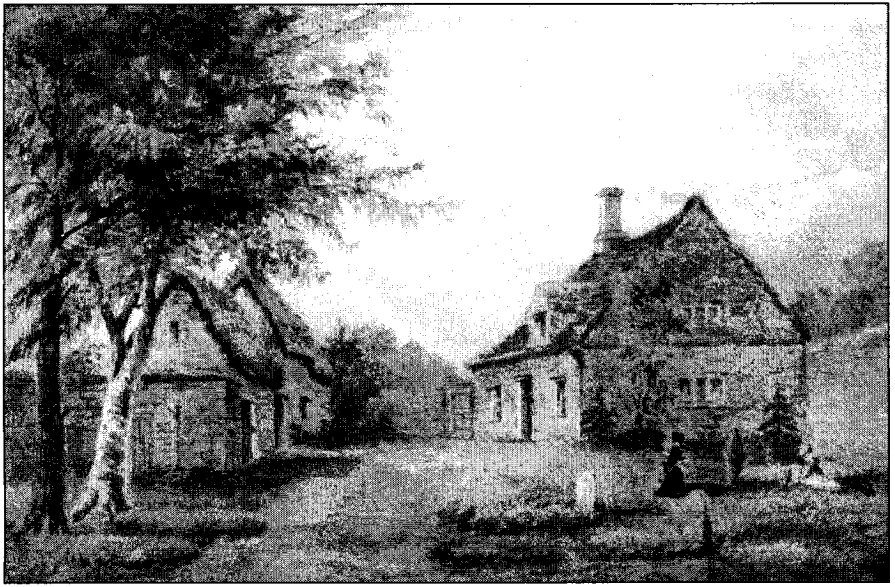
Adderbury Quaker Meeting House with attendant cottage, c.1830.
