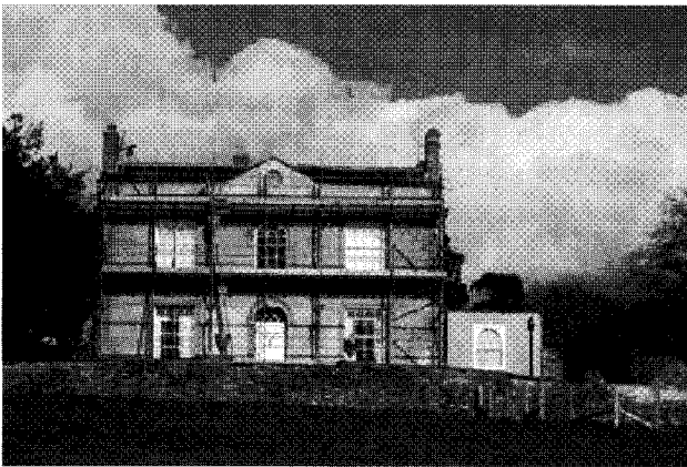
Fig 9. Holly House, Charlton, undergoing extensive refurbishment, 2009.
