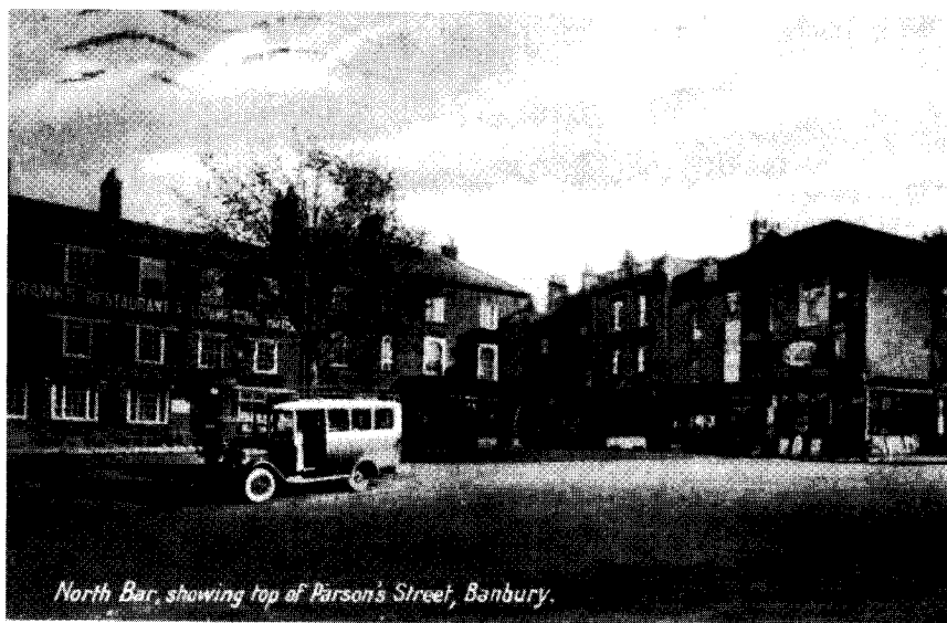
29½ Parsons Street (now 29a) is the creeper-covered first house that can be seen in the street at its junction with North Bar Street. Postcard c.1930.
