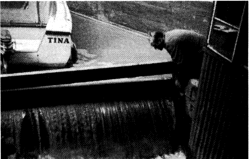
Herbert Tooley lifting the stop planks to let water into the dock.
