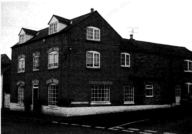
The building in its present state, with bowed windows and roof lights. The shop door is now a window; however, the brickwork at the side of the house reveals where the old wooden doors of the storeroom once were.
