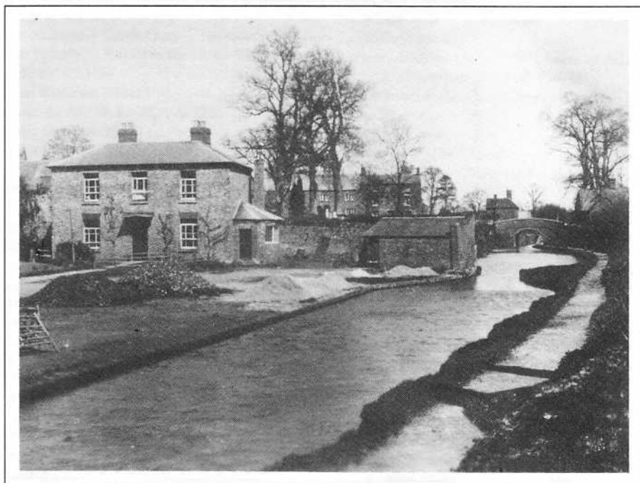
The wharfinger's house at Cropredy, with the lock keeper's house beyond the bridge, in 1926. Note the narrowing of the canal to permit checking of the boat's contents/weight (Packer's Studio, Chipping Norton).
