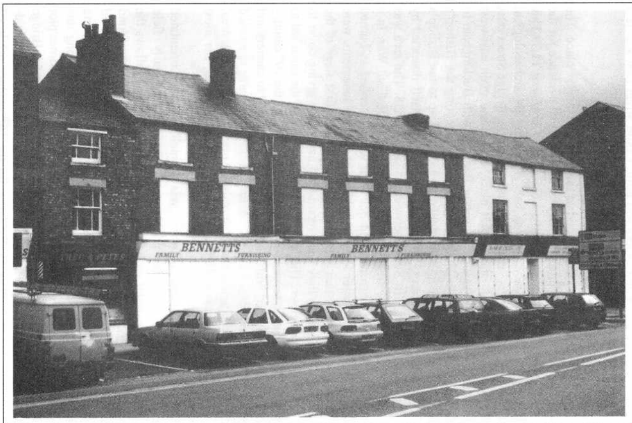
Plate 5. The facades of 53 and 54 Bridge Street.
