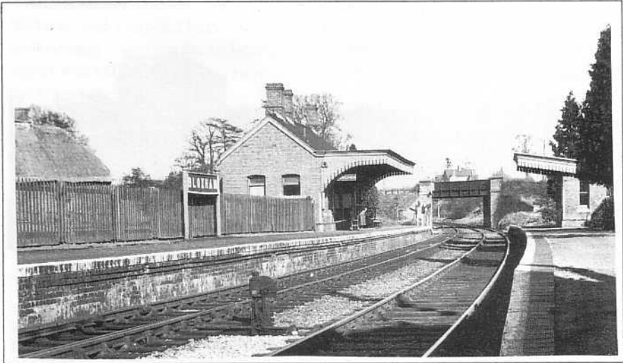
Bloxham station, located at the south-western limit of the village, looking east towards Adderbury. The Banbury and Chipping Norton road crossed the railway on the girder overbridge beyond the platform, the fourth bridge to cross the line from Adderbury within a short distance. The single line staff set down and pick-up posts (and the lamp post) can be seen at the far end of the up platform, in front of the bridge L & GRP
