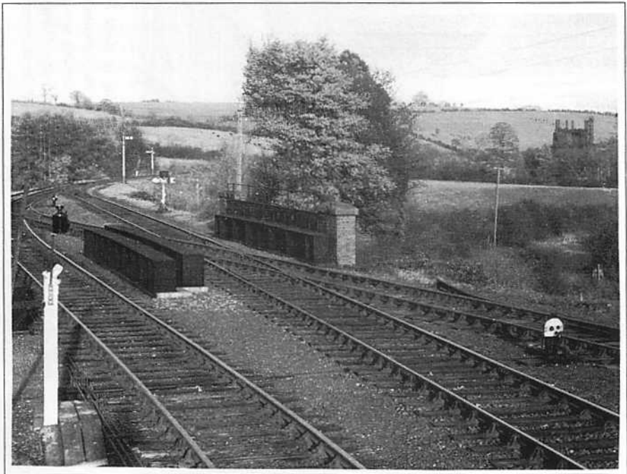
Hook Norton, looking towards Bloxham. The Brymbo kilns (at the site of Council Hill Sidings) can be seen on the right, just under a mile from Hook Norton station. SRM/JHR
