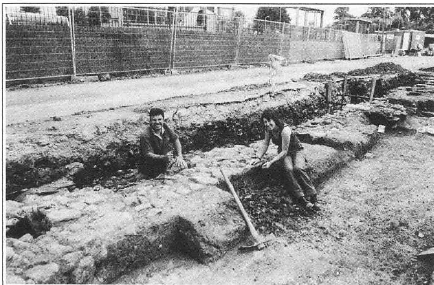
Plate 3. Medieval building foundation, Mill Lane.
