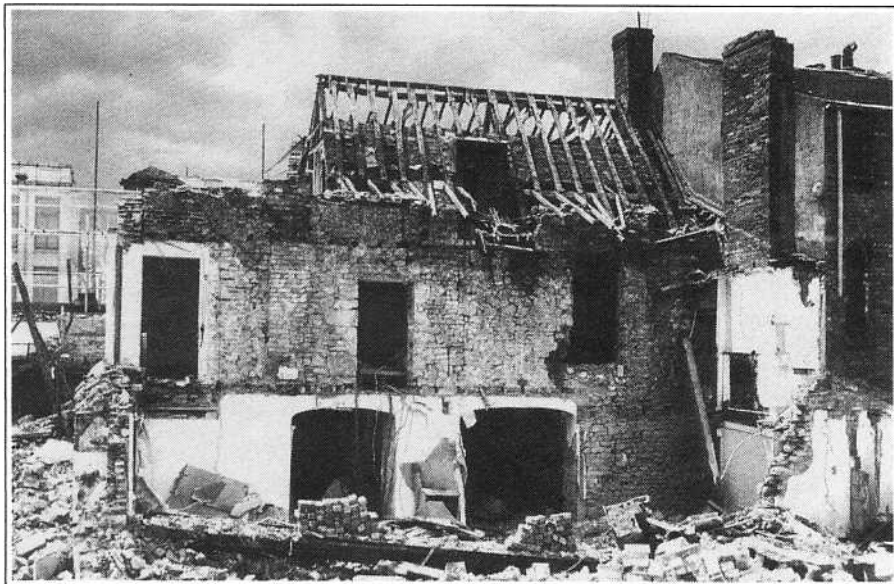
Plate 2. Survival of ironstone building and early roof structure, 54 Bridge Street.
