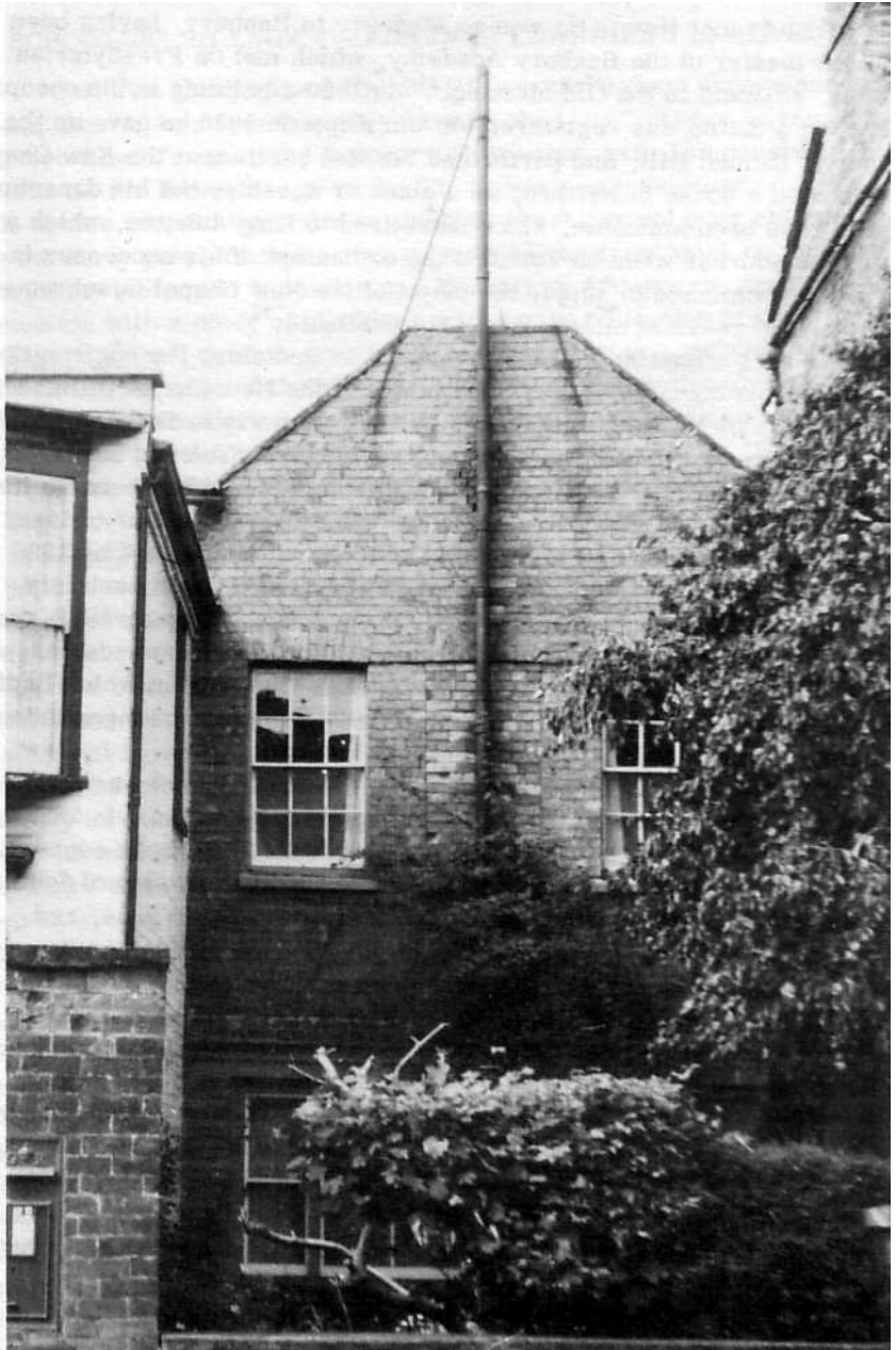
No.34b West Bar, Banbury, demolished in 1969, between 1829 and 1877 this was the chapel used by the Gardner family's Calvinistic Baptist Congregation. After Banbury's streets were first numbered in the 1850s it was known as 17½ West Bar.
