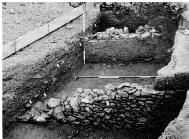
Plate 1. First phase of castle building – looking east.
