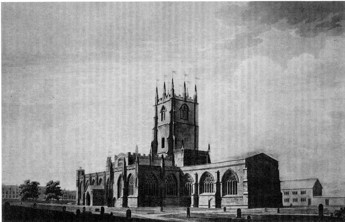
Figure 1. St. Mary's, Banbury: The old church, viewed from the south-east. A drawing by John Wells. (Bodleian Library, Oxford).
