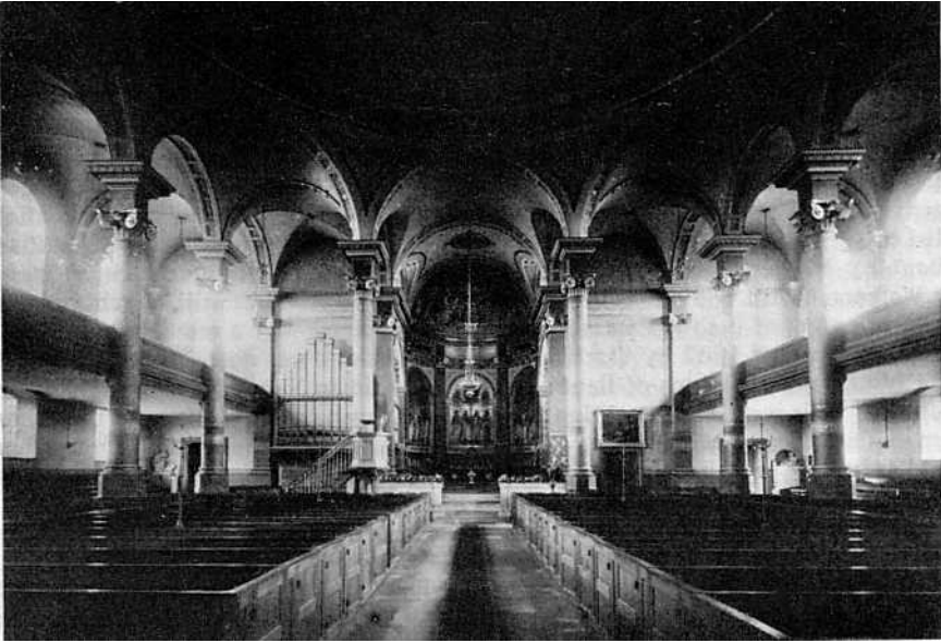
Figure 8. St. Mary's, Banbury: the interior looking east in about 1890, photographed by H. Taunt, showing the chancel as altered by Blomfield, with its steps and imitation mosaic paintings, the new and repositioned pulpit, and the rebuilt organ case. (Oxford Public Libraries, CC72/385, and National Monuments Record).
