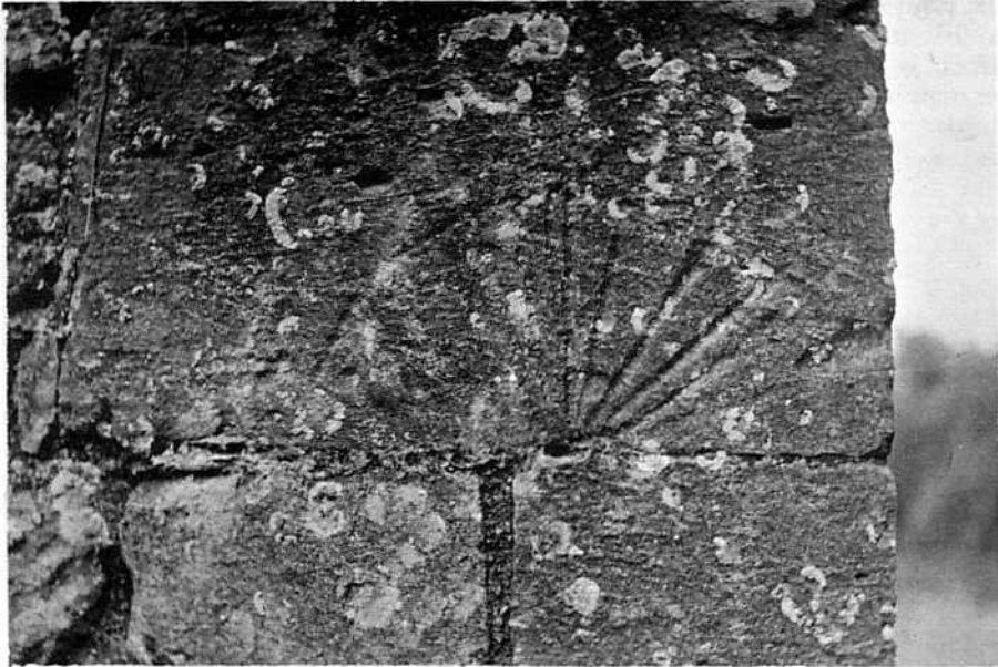
Figure 5. Inverted dial, resulting from disturbance of stones during restoration. Tackley, Oxon.
